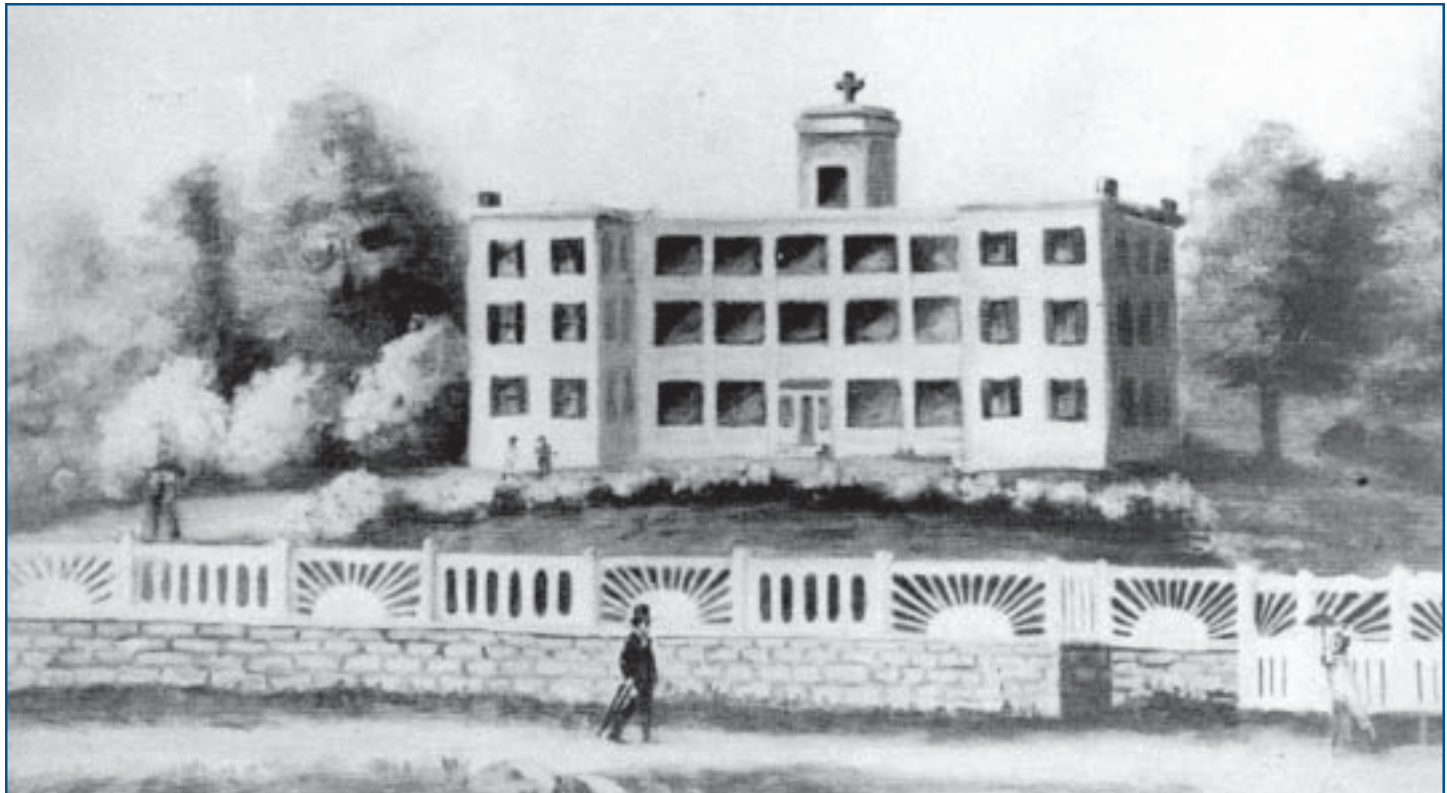
The first motherhouse of the Sisters of Charity of New York – Mount Saint Vincent at McGown's Pass – opened in 1847. This site is now within Central Park at approximately 105th St. & Fifth Avenue.
